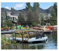
This dock (left) does not have a section fixed to the shore and has only one set of piers into the ground with two support pillars which impacts the entire dock's horizontal stability. In addition to this dock, there are others on the East side of the lake with a similar two pillar design.
